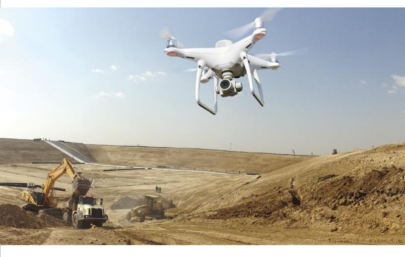
The GNSS data files are post processed, and time stamps (event markers) are used to accurately geotag the images.
