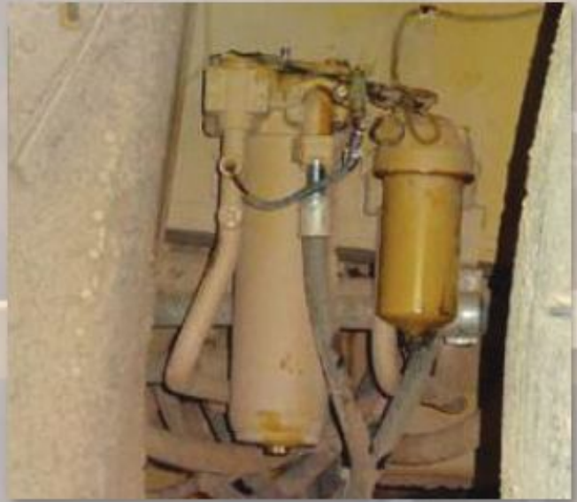
Transmission Charging filter canister (left).
